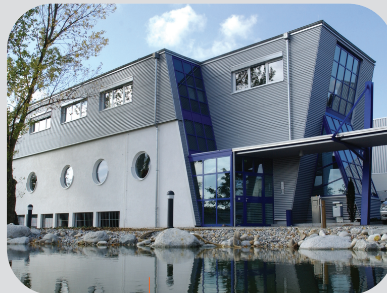
In 2001, Aero Pump constructed a new building in Hochheim, Germany.
